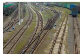
Rail Shunting Lines Outgoing Hausmann Bromelton Plant Rail Systems
