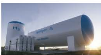
Hausmann Bromelton Gas Power Plant
