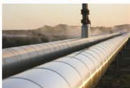
Gas Pipeline Construction (37km) from Ipswich to Bromelton
