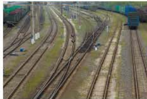
Rail Shunting Lines Incoming Hausmann Bromelton Plant Rail Systems
