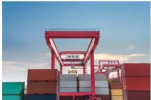
Deep Water Port Facility (if applicable)
